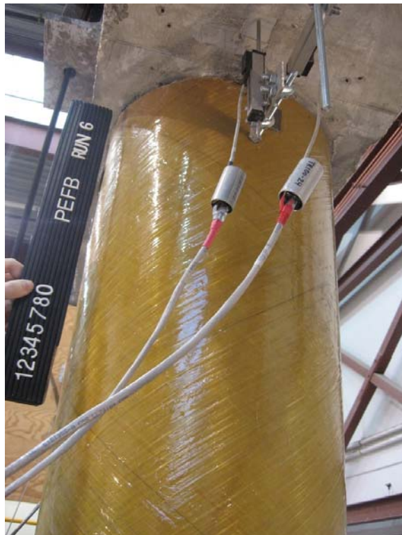
a) FRP Column, North, Run-6
