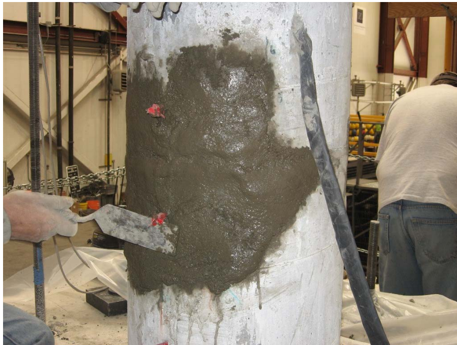
Fig. 2-53. Patching SC-2R with High Strength Grout
