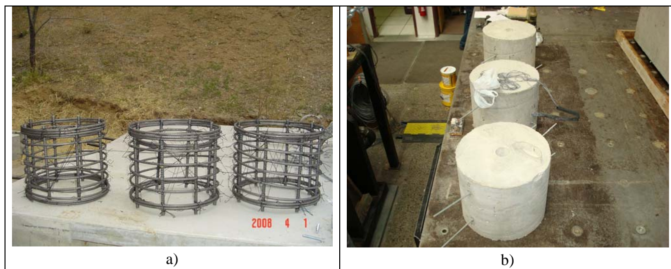
Fig. 2-27. Typical Segments, a) Steel Cages, b) after Construction
