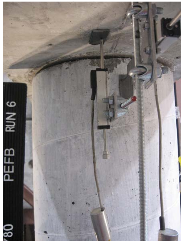
b) RC-ECC Column, South, Run-6
