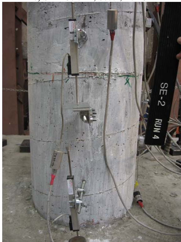
d) SE-2 Column, South, Run-4
