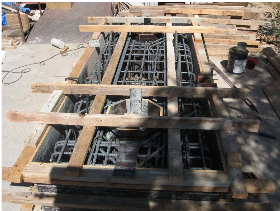
Fig. 2-71. PEFB Footing before Casting of Concrete
