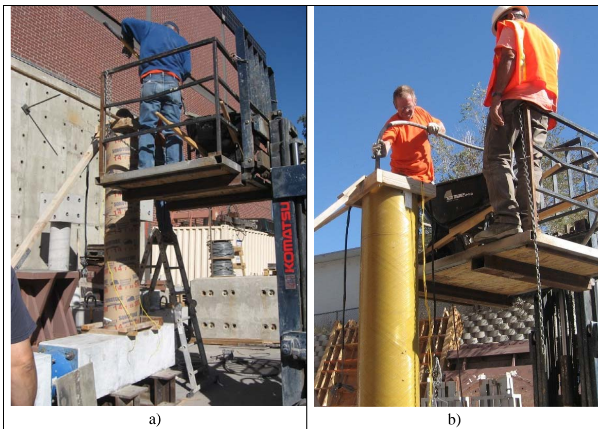
Fig. 2-73. PEFB Columns Concrete Casting, a) RC-ECC Column, b) FRP Tube
