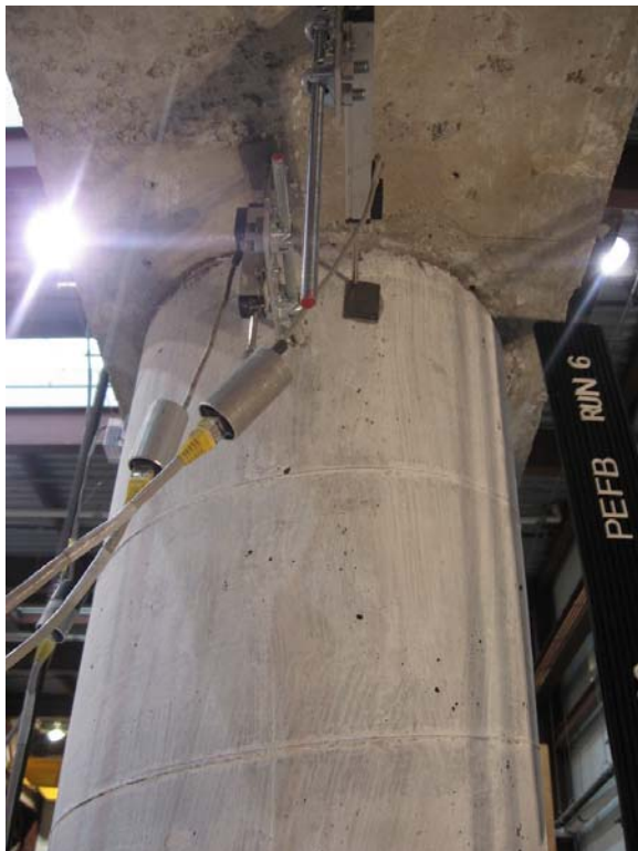
a) RC-ECC Column, North, Run-6
