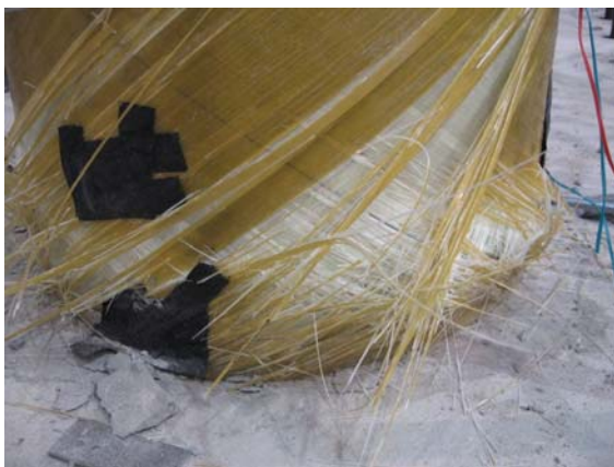
a) FRP Rupture, South, Run 6
