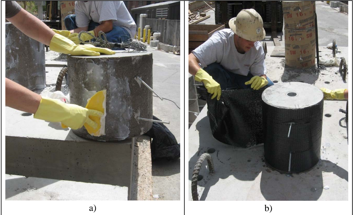
Fig. 2-40. a) Preparing the Surface, b) FRP Wrapping
