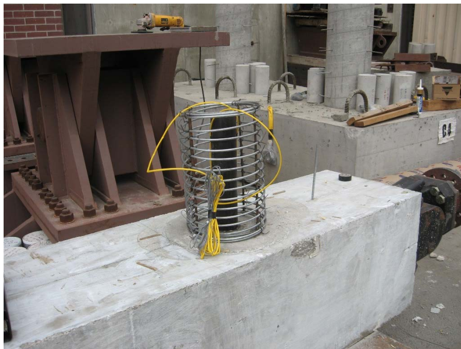
Fig. 2-69. Setting Up Pipe-Pin Hinge Detail on the Cap Beam
