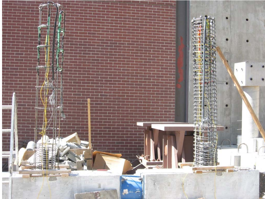
Fig. 2-70. Setting Up the Column Cages on the Cap Beam, Up-Side-Down Construction
