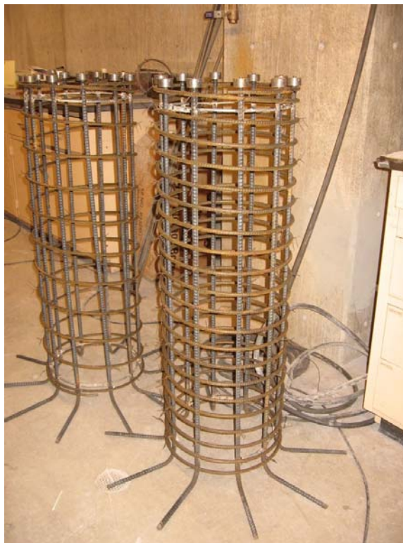
Fig. 2-16. Base Segment Steel Cage
