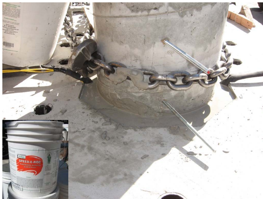
Fig. 2-78. Filling the Opening with Fast Setting Grout
