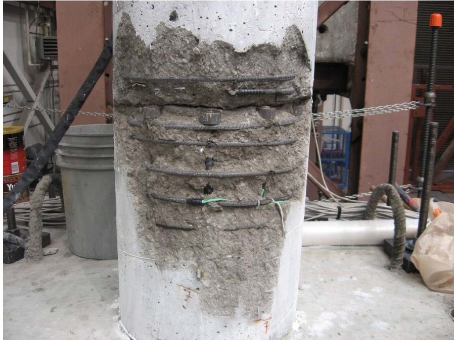
Fig. 2-52. SC-2R Repair Process, Removing Loose Concrete
