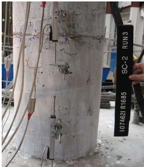
a) SC-2 Column, North, Run-3
