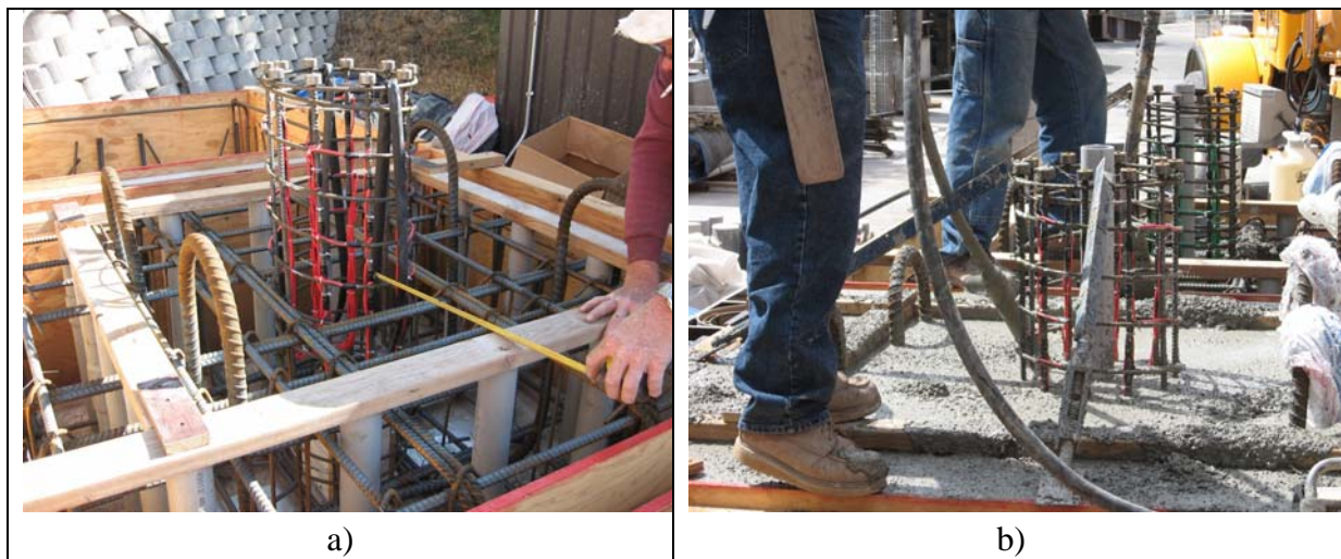
Fig. 2-38. SF-2 Footing and Base Segment, a) Before Casting, b) After Casting
