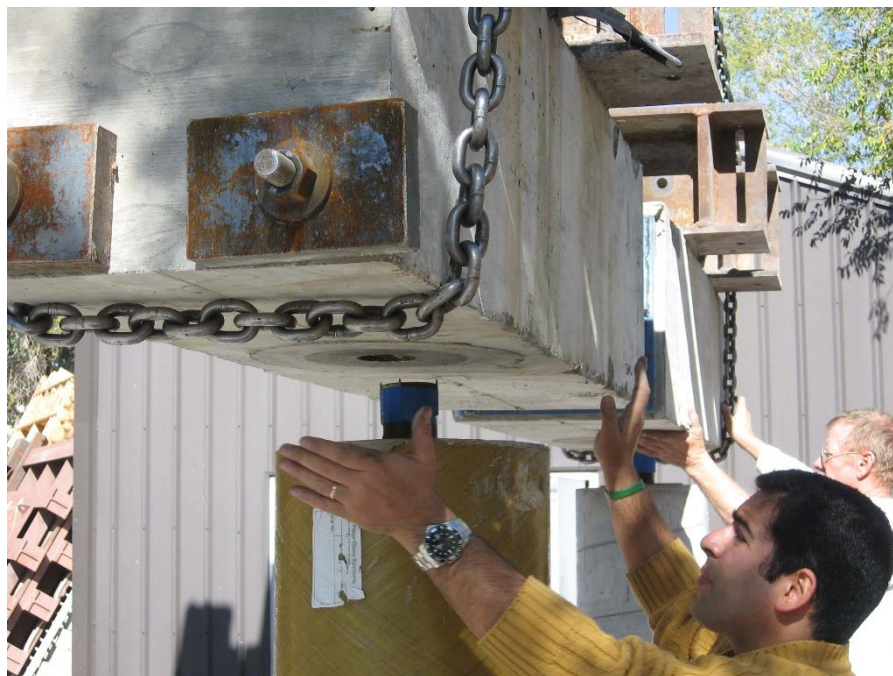
Fig. 2-77. Cap Beam Installation
