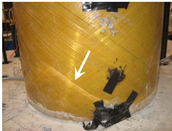
b) FRP Buckling, North, Run 6
