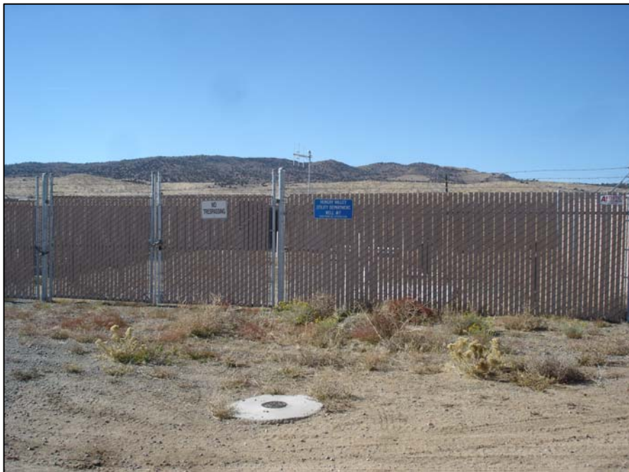
Figure 20. Well No. 7 (Enclosure)
