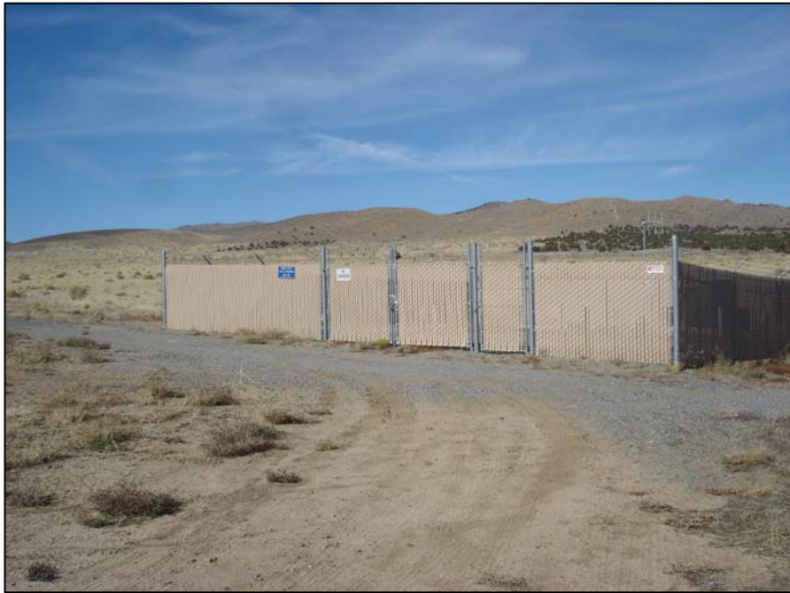
Figure 22. Well No. 8 (Enclosure)
