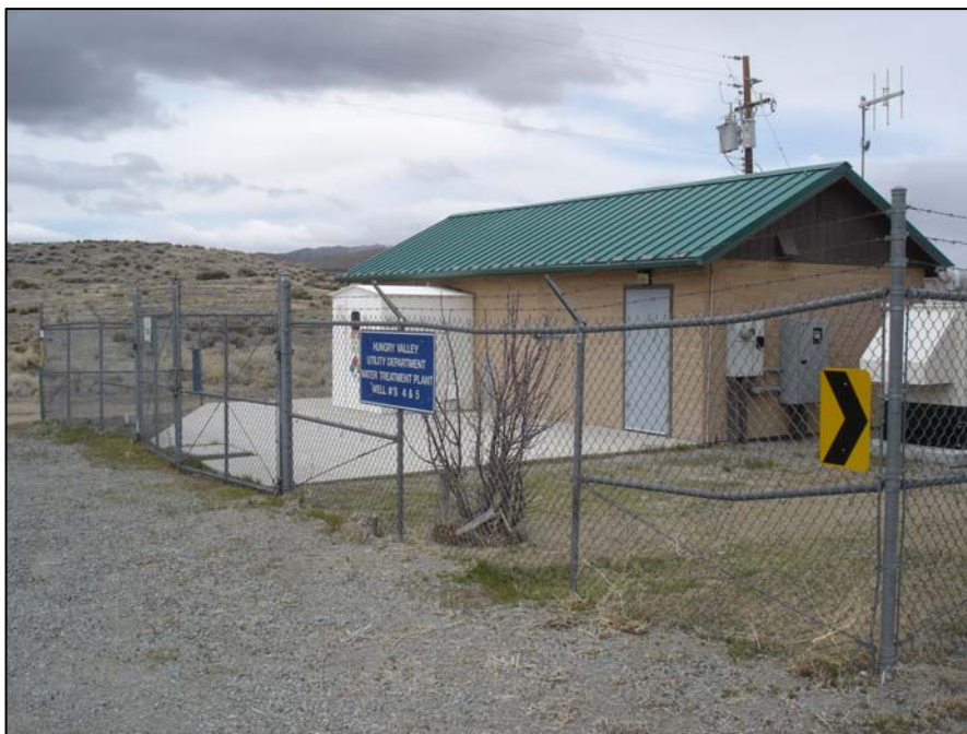
Figure 27. Hungry Valley Utility Department, Water Treatment Plant
