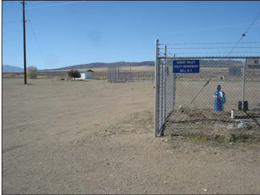
Figure 17. Well No. 3 (w/RSIC Air Station in the Background)
