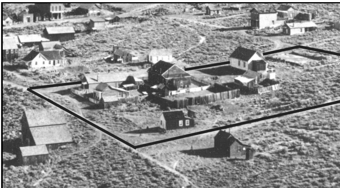
Figure 2. The back of the Levy and Kaufman residences as seen from Lover's Leap, 1890. Block C is outlined in black. Photo courtesy of the Nevada Historical Society and Cliff Shaw.
