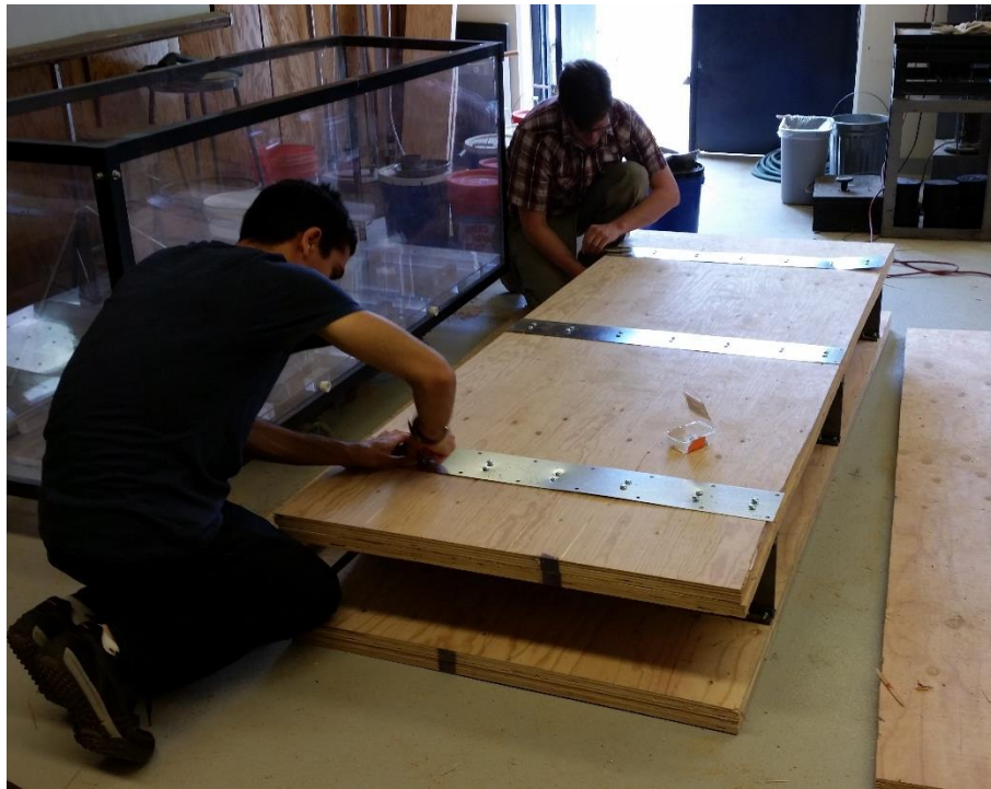
Figure 3-4: Construction of top half of Shake Table
