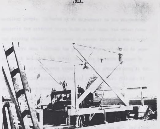
Fig. 35. Type of moving screen that has proved very satisfactory for cleaning water before pump intake.
