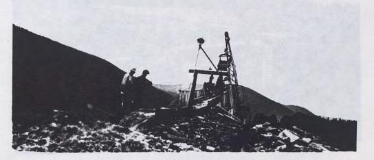
Fig. 28. Sluice with 5 sections of tailings boxes in place.
