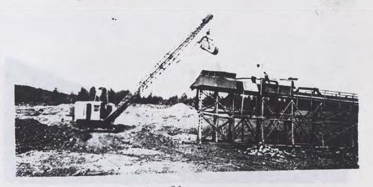
Fig. 26. Dragline in operation. Note the way the Bulldozer has cleaned the bedrock in front of the dragline.
