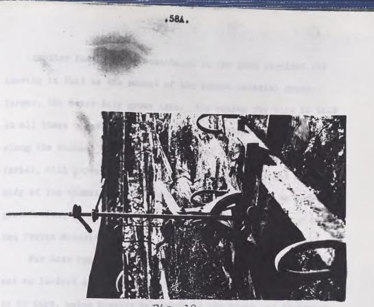
Fig. 19. Foint pulling clamp with wrenches used for pulling points when ground is thawed. Note the large base used to keep the clamp from sinking into the soft ground.
