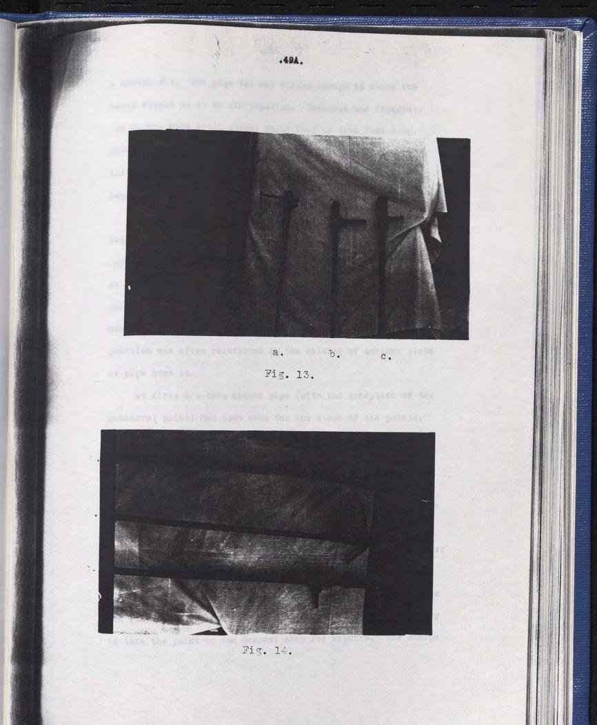
a shrink fit. The pipe was not strong enough to stand the heavy strain on it at the junction. Breakage was frequent. The points were still short, about four to five feet long. Later the bottle neck was developed. This type of neck distributed the strain on the junction between pipe and head. The nipple point is illustrated in Fig. 14, a.
