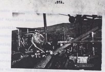
Fig. 49. Carrier and bucket, used in drift mining.
