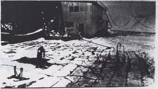
Fig. 57. Thewing ice with storn Note method of holding U in place so one mon can keep several thaws going at one time.
