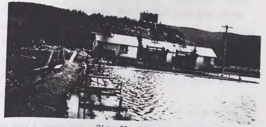
Fig. 21. 3 - 5000 gallon per minute pumps. Note screens for cleaning intake water so the small hole on the bottom of the thaw point will not be plugged. Dam for pond is on the readers left.
