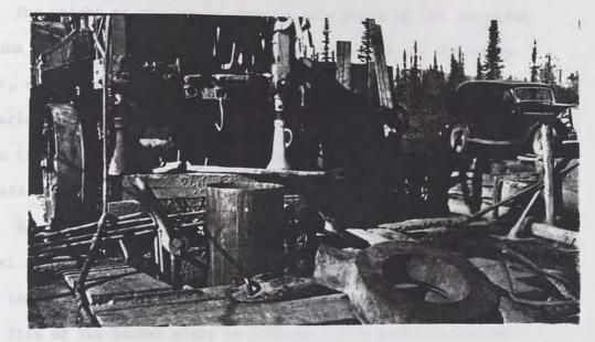
Fig. 54. Keystone drill used for sinking an 18 inch hole to bedrock. Depth of hole 240 feet. 18 inch casing pulled into hole with the aid of hydraulic jacks.
