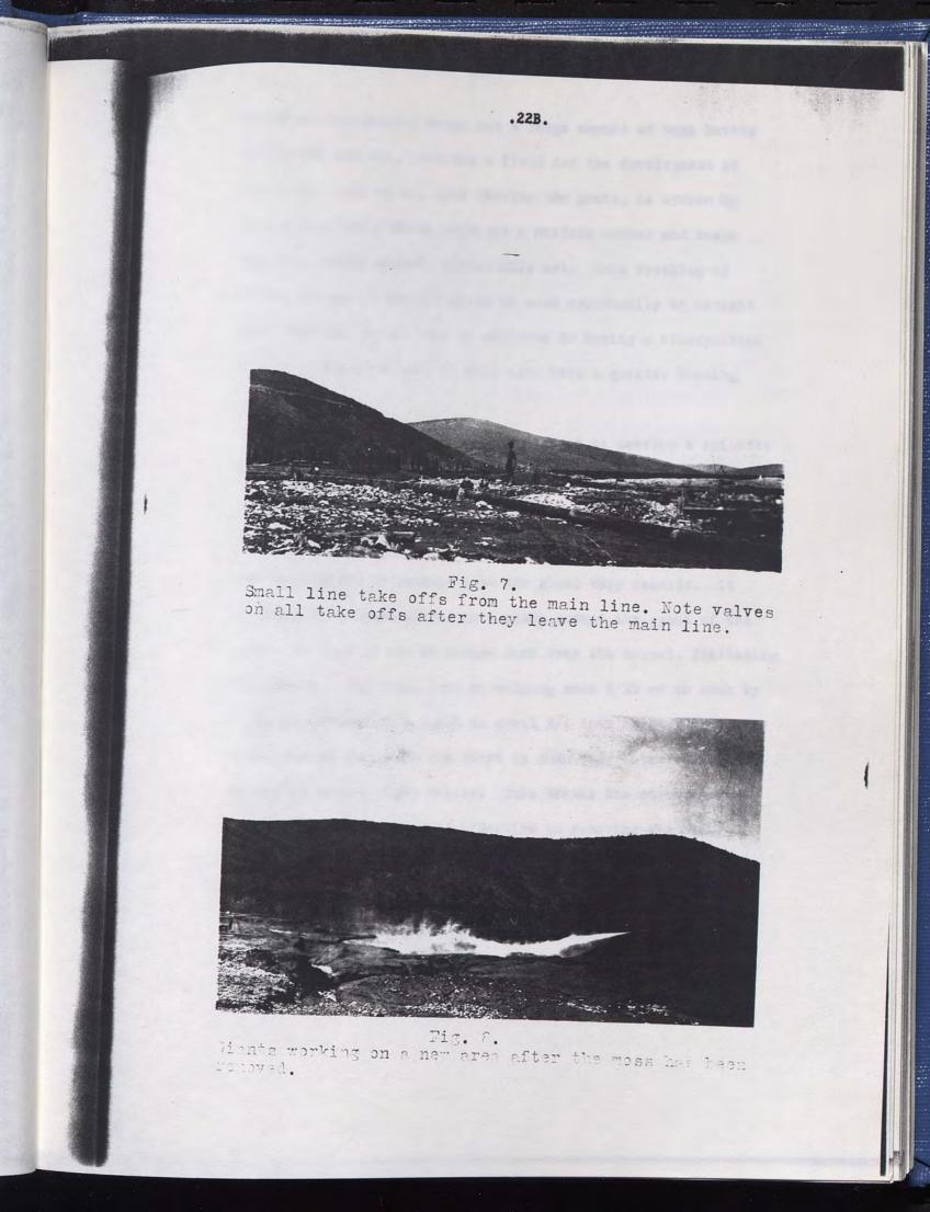
excess of inexpensive water and a large amount of muck having a high ice content, provides a field for the development of the spray. The water, upon leaving the giant, is broken up into a fine spray which provides a uniform shower and keeps the area, being worked, continually wet. This breaking-up of the stream in the air gives it more opportunity to extract heat from the air so that in addition to having a transporting effect on the muck bed, it will also have a greater thawing effect.
